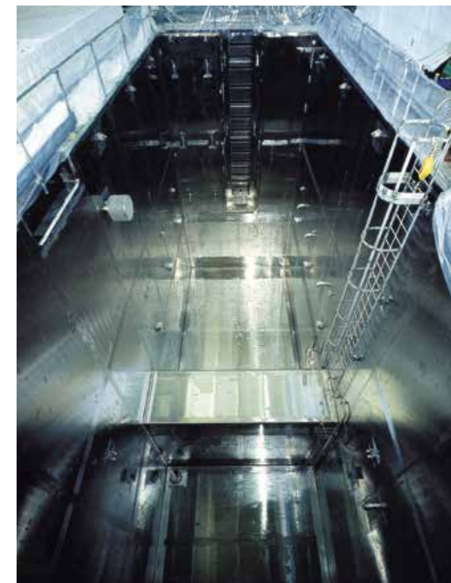
Stainless lining at nuclear energy plant
